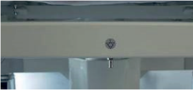
Fig. Potential equalisation connector – male
